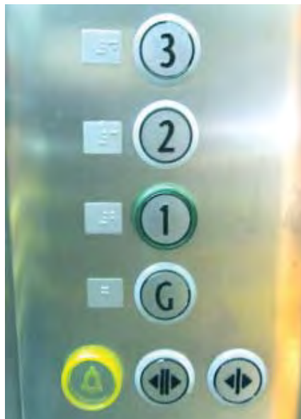
Door-hold push button alongside door-open push button
