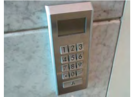
Keypad-type landing registration terminal
