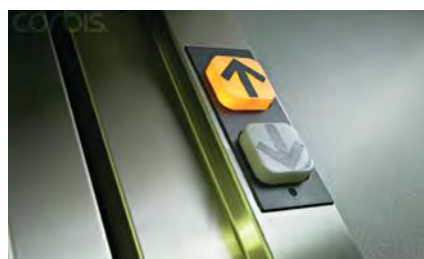
Car lantern installed on the elevator's entrance column
